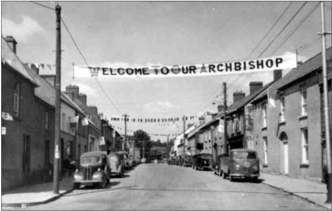
View of Upper Main Street on this special occasion.
