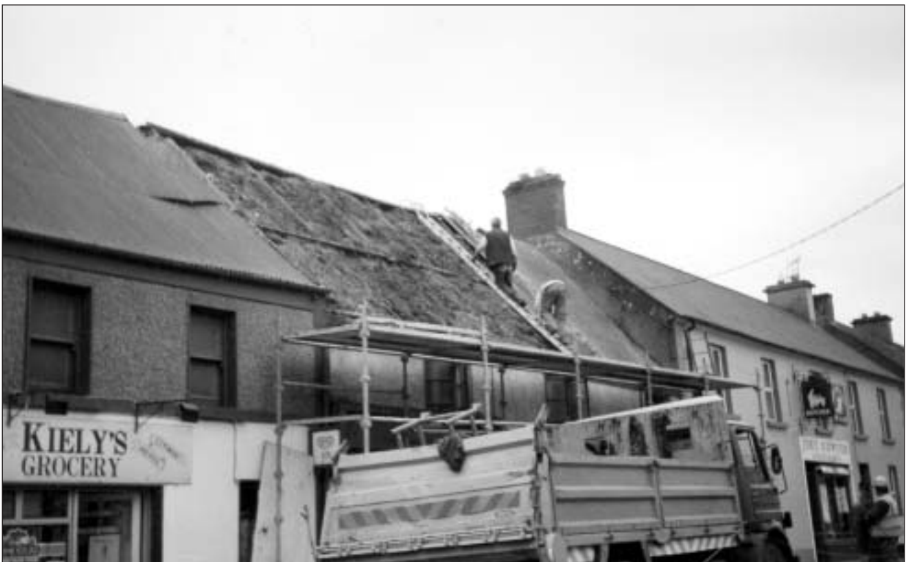
Mary Smith's shop being demolished to make way for the new carpark.
